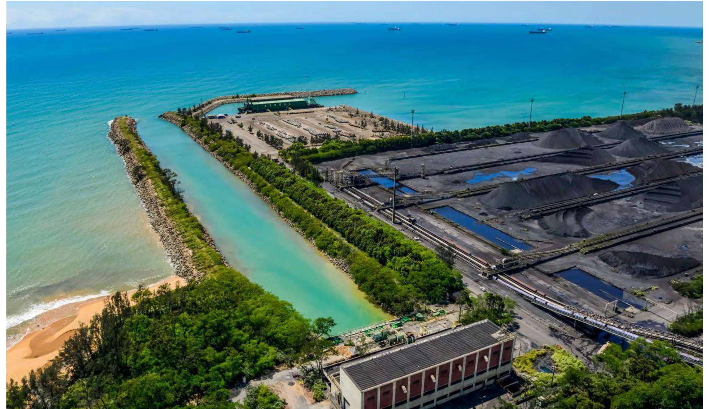
Desalination Plant, located at the Tubarão Unit, in the State of Espírito Santo
